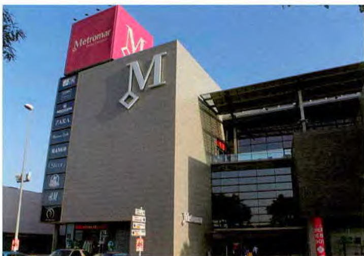
Metromar Shopping Center, Seville
